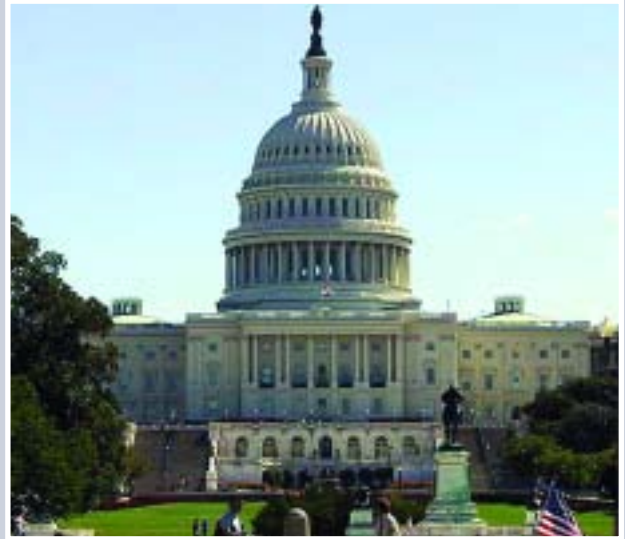
[illus. 11] U. S. Capitol in Washington D.C. showing the new dome and side wings, designed by Thomas U. Walter
